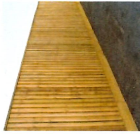
Lapped & capped timber fence
